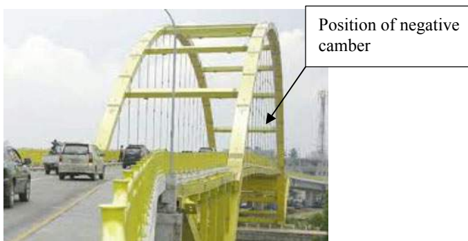
Fig. 1 Visual observation arch steel bridge of Siak III bridge
