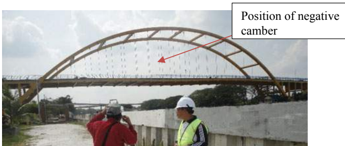
Fig. 3 Measuring camber position bridges with total station
