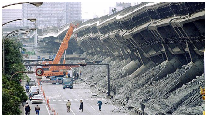
Fig.1 Higashi-Nada Viaduct collapse in 1995 due to Kobe earthquake [3]
