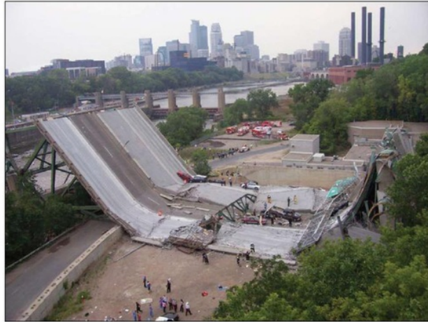
Figure 1. One section of the I-35W Bridge collapse [6]
