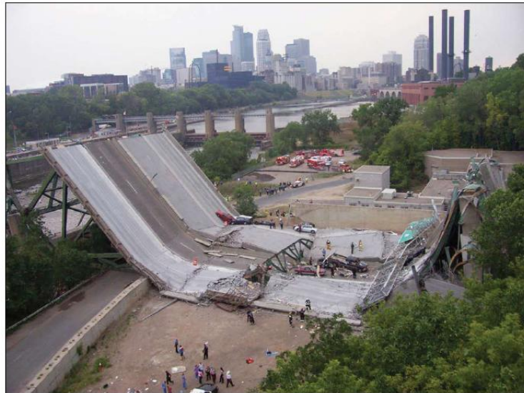
Figure 1. One section of the I-35W Bridge collapse [6]
