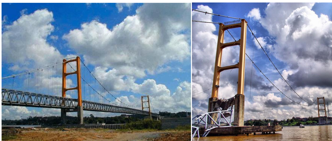
Figure 2. Kutai Kartanegara Bridge before and after collapse [7]
