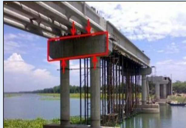
Deep beams as transfer girder
