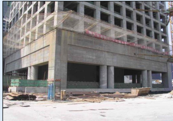
Deep beams as transfer girder
