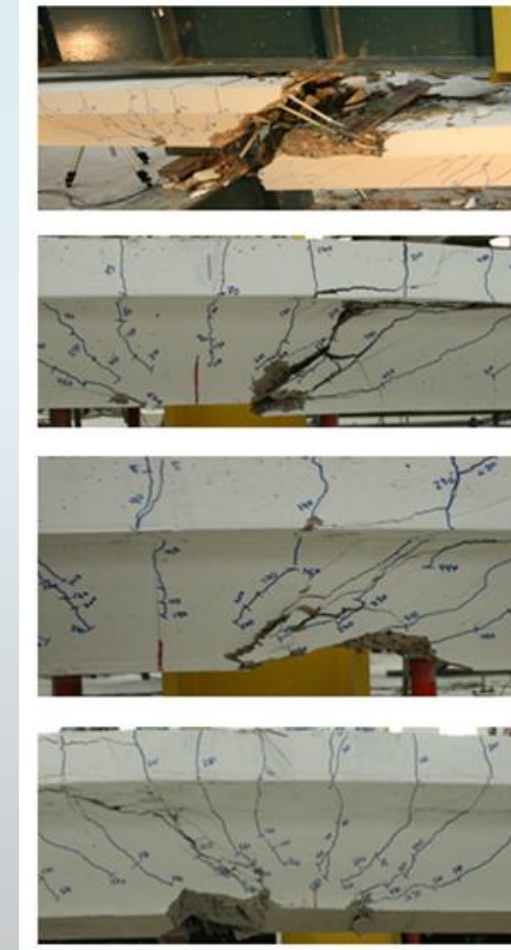
Observed mode of failure
