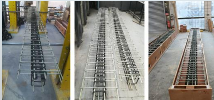
2. Preparation of the reinforcement cages.
