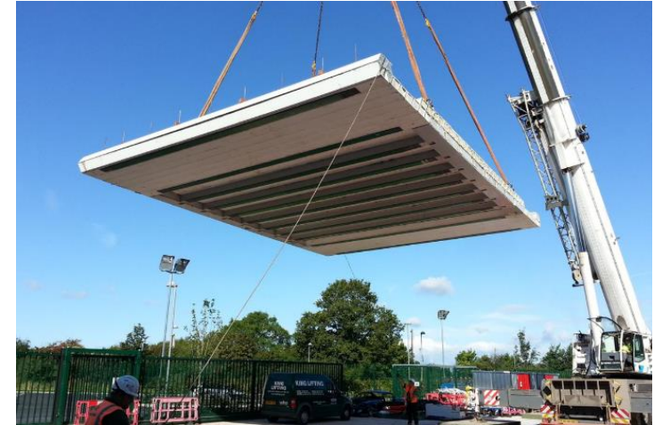
Church Lane Bridge
